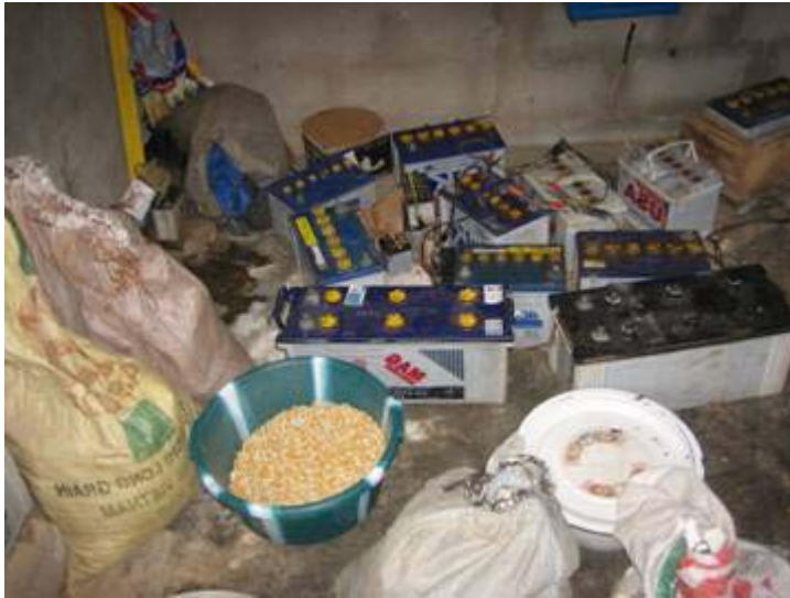
Batteries for charging in Koumantou, Mali
