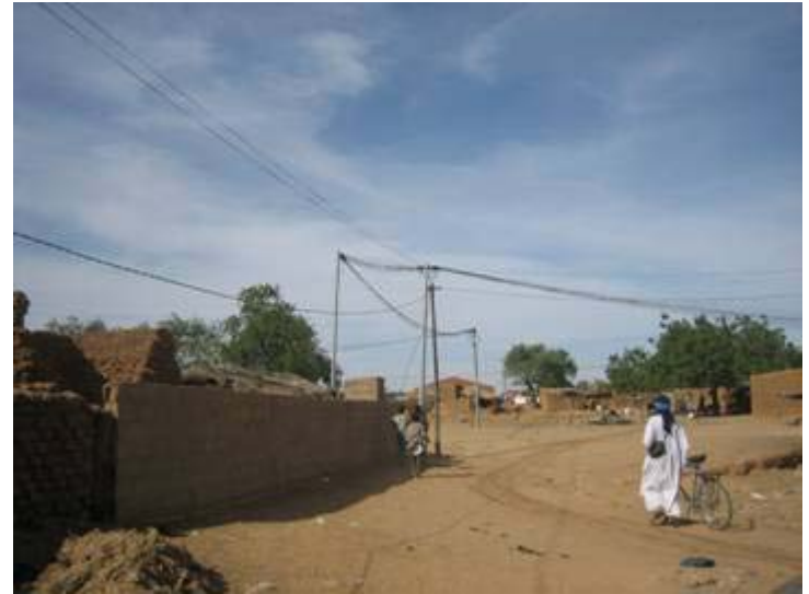
Electricity wires in Sebba, Burkina Faso
